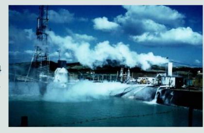
Top: Geothermal pilot plant production test C1 well (1981-82) [Source: STEAM 2023] Bottom: Some of the C1 pipe work showing natural precipitation of minerals (scale) from brine [Source: STEAM June 2023]
